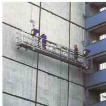
Suspended working platforms
