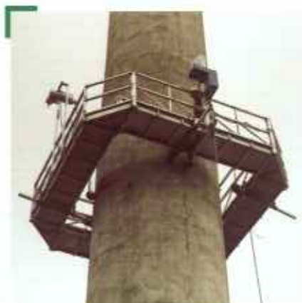
The platform can be adjusted to the shape of the building using corner sections.
