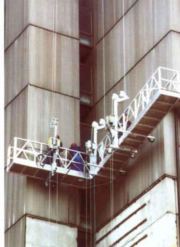
By means of special controls up to 4 drive units can be operated simultaneously allowing to use also larger platform assemblies.
