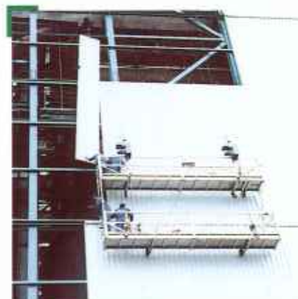
For the installation of curtain wall panels the double-deck version is often used to allow fixing of the panels at the same time at several places.
