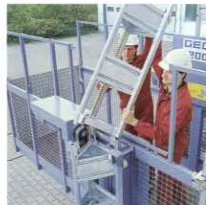
Comfortable assembly of the 1.5 m high steel mast sections (hot-dip galvanised) with captive screws and nuts.
