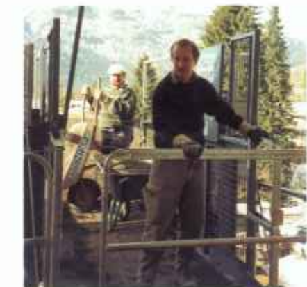
Hot-dip galvanised landing level safety gates (1 piece is supplied with the base unit) with mechanically locked sliding door are installed at the landing levels to ensure safety of people.
