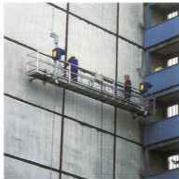
Suspended working platforms
