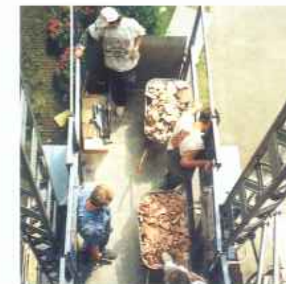
The load platform has a lot of space for bulky and heavy materials. Load platform variant "B", dimensions 1.45 x 3.3 m.
