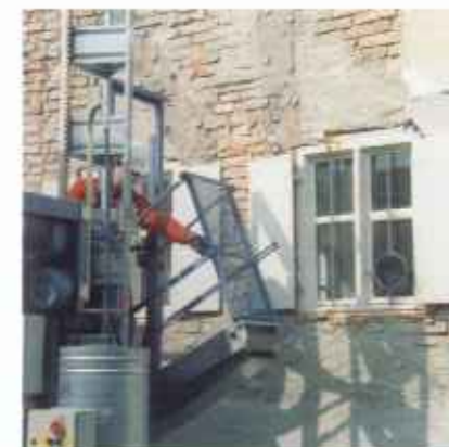
Assembly plank (can be retrofitted) for anchoring the transport platform without pre-built scaffold.
